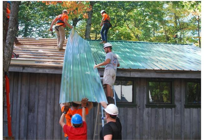
Thanks to our Davis grant, we were able to get a new roof on the old Lombard shed. UM Construction Management Technology students put the funds to use, did some rafter work (some had been cut to allow the Lombard space!), and the metal roof went on very quickly. Trim and paint are on the list for this summer.
