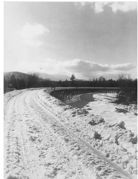
Great Northern Paper Company's 1,250 foot long Cooper Brook log hauler trestle Circa 1928. Terence F. Harper Collection
