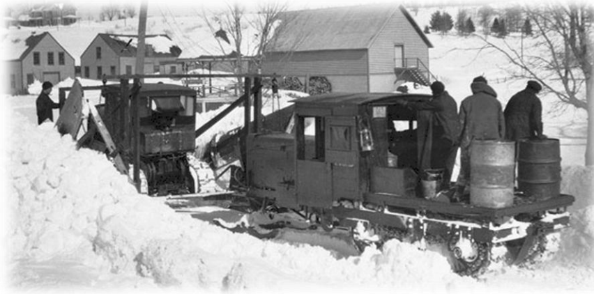
Great Northern paper Company 10 ton Lombard tractor and Holt crawler breaking open a road. Terence F. Harper Collection
