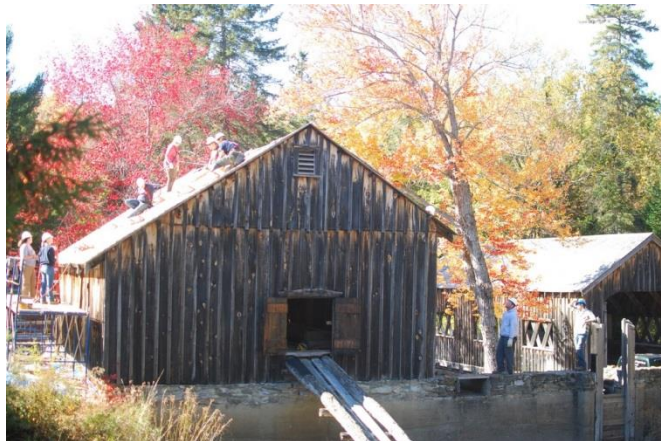
Shingling water-powered sawmill roof
