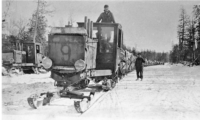
Lacroix's fleet of 10 ton Lombard tractors ran 24 hours per day, 6 days per week moving pulpwood from as far away as the Musquecook Lakes to Churchill Lake.
