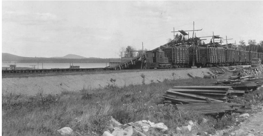
The Plymouth locomotive spots cars under the loading conveyors at Tramway. Terence F. Harper Collection
