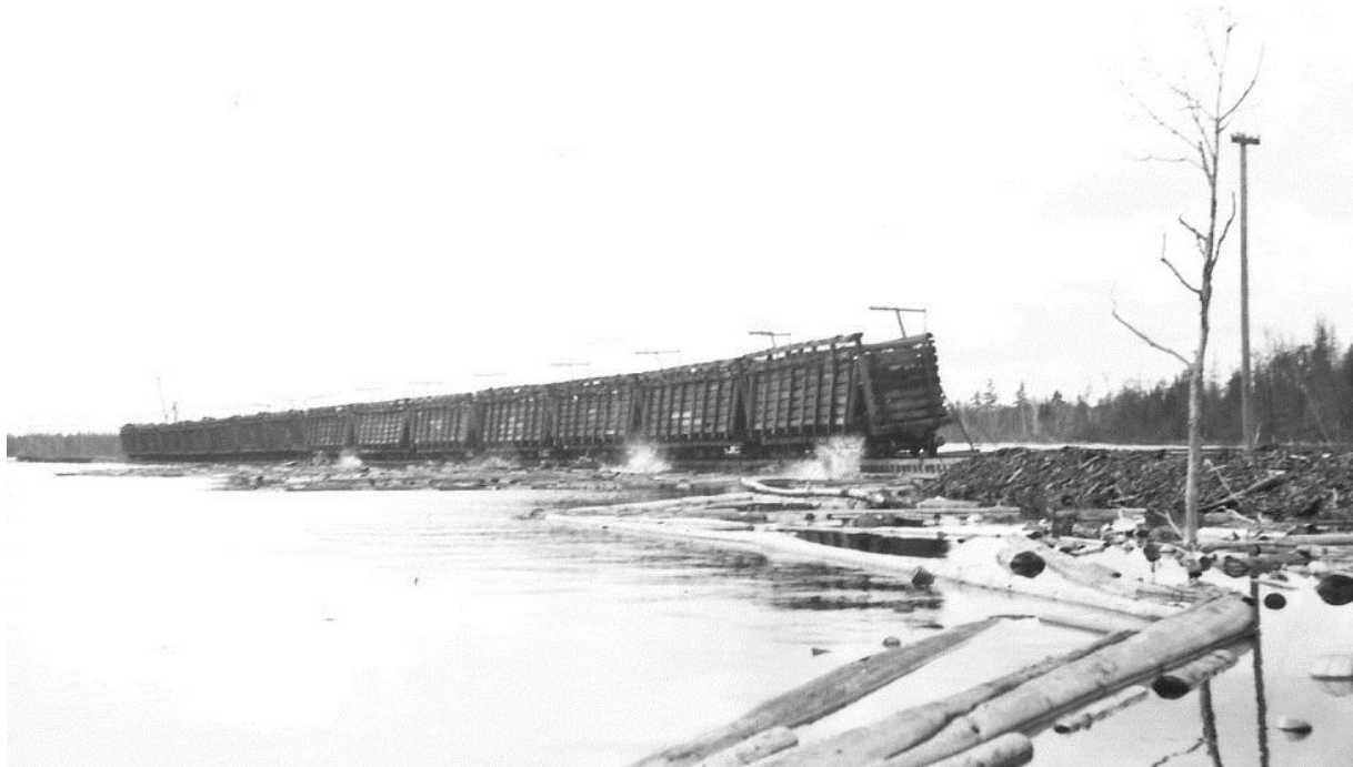
With one rail of the unloading trestle set 6-inches higher than the other and in combination of a sloped floor, most of the pulpwood tumbled out when the door was unlatched.
