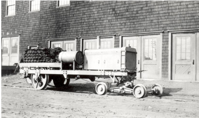
The EL&WB rail truck was a Lombard 10-ton tractor converted to run on rails. Note the logs stacked on the back platform. This photo was taken at the Lombard factory in Waterville, ME.
