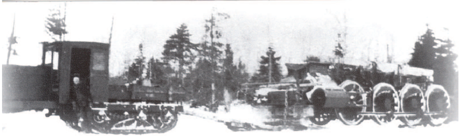
Above: The frame of EL&BW #2 heads for Tramway behind a Lombard tractor. After arriving at Lac Frontiere, Quebec, both of the EL&BW's steam locomotives were disassembled and mounted on sleds for the 50-mile trip through the wilderness.
