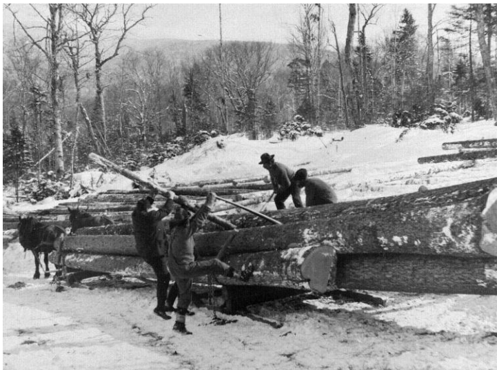
Loading a sled was a backbreaking and dangerous job. Corner chains bind the bottom outside logs to the bunk with deck chains holding the stakes firm against the load. One or two wrapper chains secure the upper logs to the lower logs - often using a spring-pole to tighten the chain.
