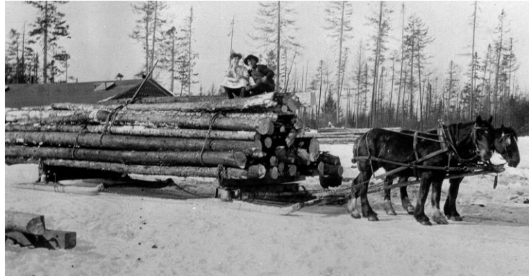
For over 80 years the "Two-Sled" rig was the primary means of hauling logs from the cuttings to the landings.
